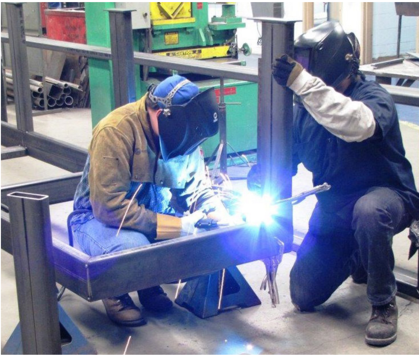
Students in Welding and Auto Collision collaborate to build ramps for the Locomotive Diesel Technology pathway.
